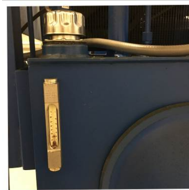
Figure 5. Sump Tank Sight Glass
