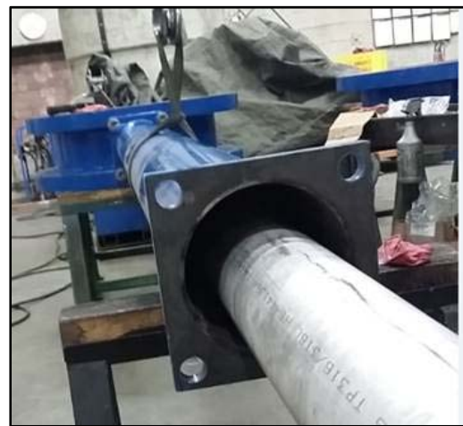
FIGURE 5. INSTALLING OUTER SHAFT
