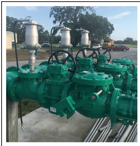
Single Body Wastewater Combination Air Valve
