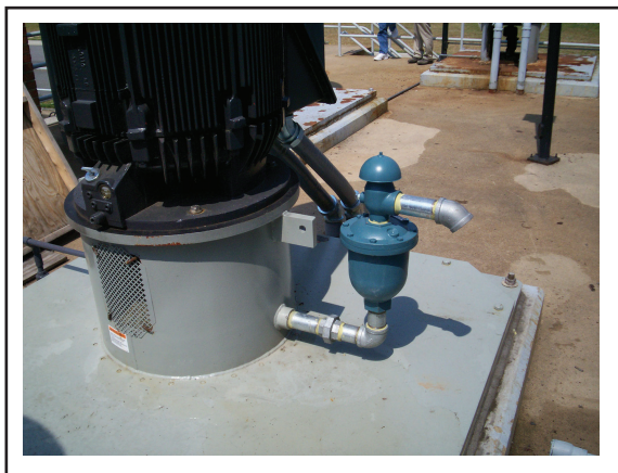
Air/Vacuum Valve with Dual Port Throttling Device
