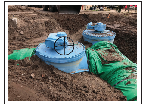
Cam-Centric® Plug Valve with worm gear actuator
