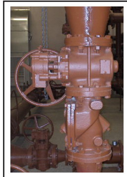
Cam-Centric® Plug Valve with Val-Matic Swing-Flex®
