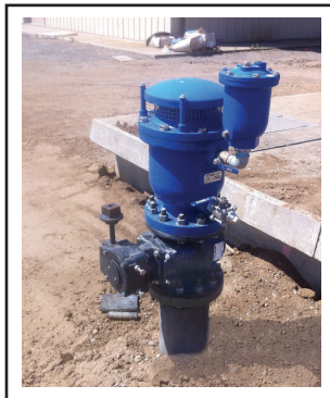
Cam-Centric® Plug Valve with Val-Matic dual body combination Air Valve
