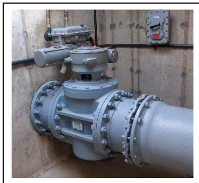
Cam-Centric® Plug Valve with motor actuator
